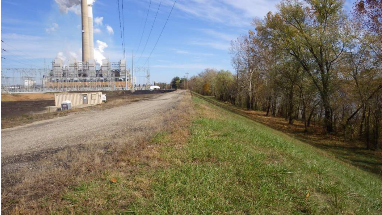
Photograph 13 – Downstream eastern embankment of BSP.
