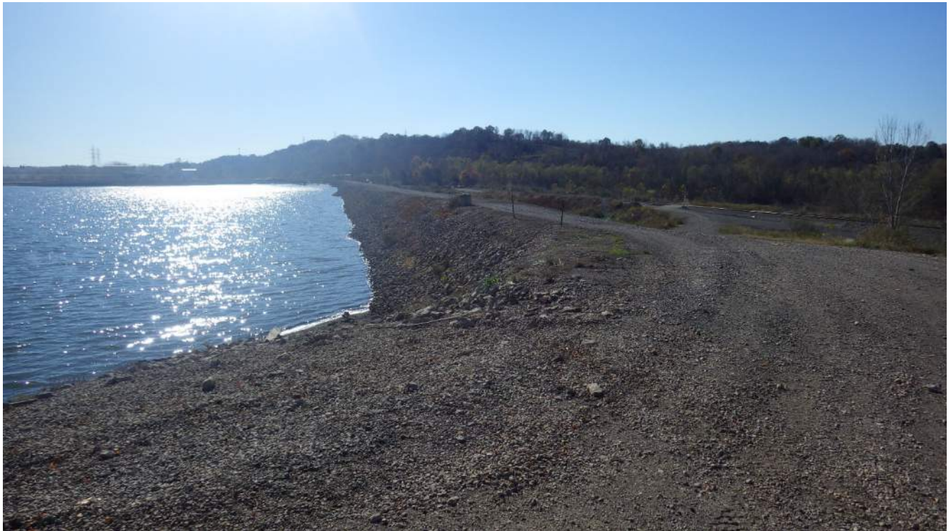
Photograph 12 – Western embankment showing upstream riprap protection.
