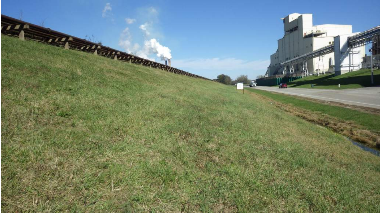
Photograph 5 – Downstream side of eastern perimeter embankment.
