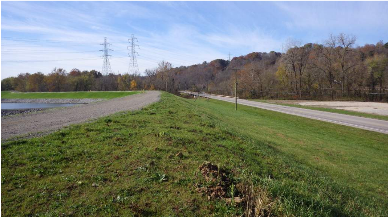
Photograph 2 – Western embankment of BSP.
