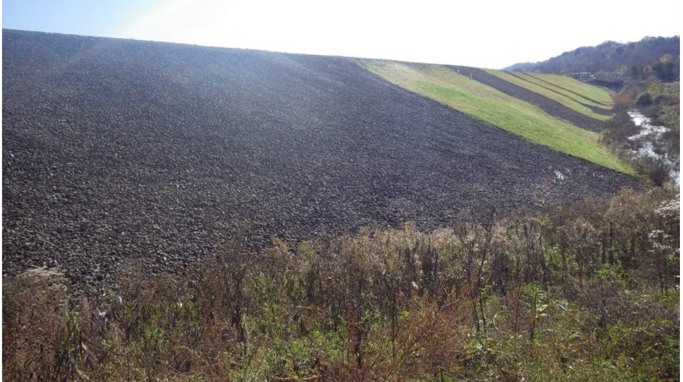
Photograph 13 – Aggregate seepage blankets on western slope.
