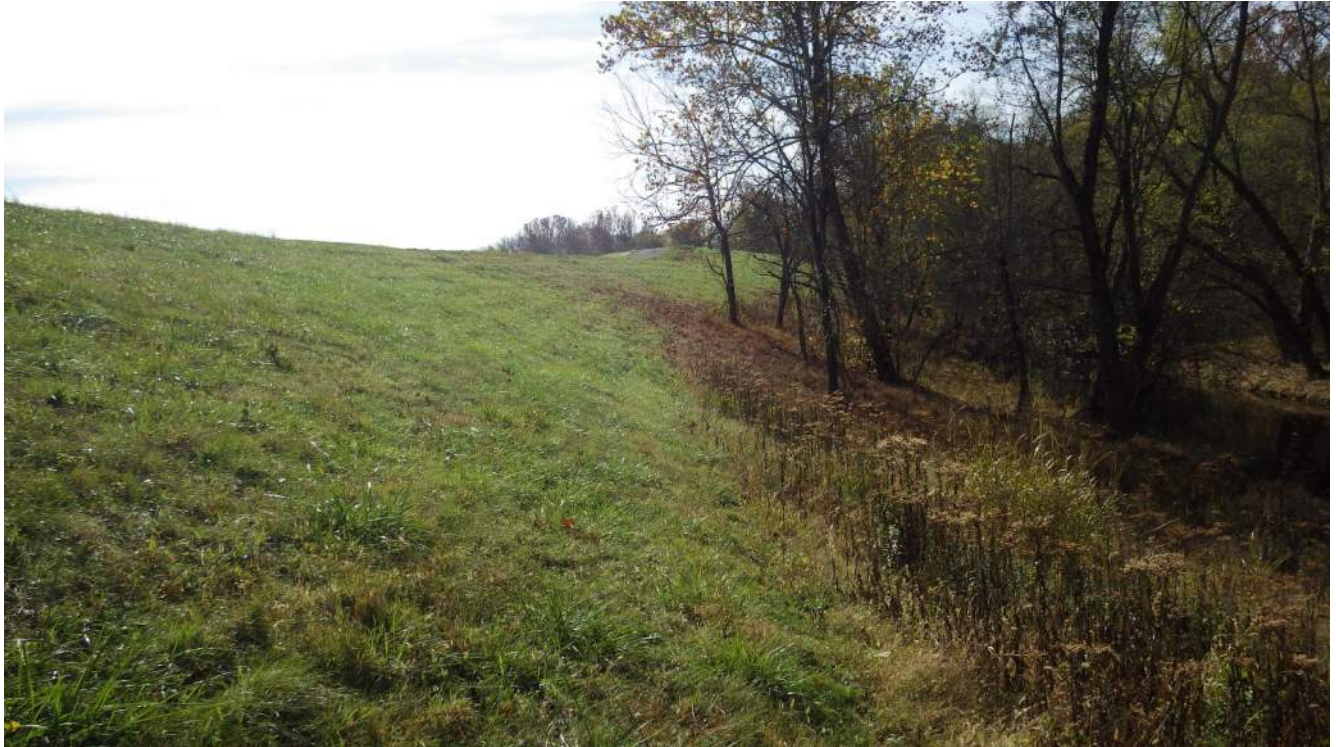
Photograph 7 – Downstream southwestern slope near Kyger Creek.
