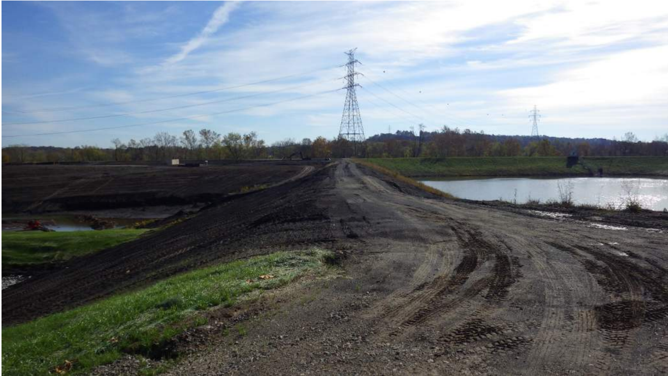
Photograph 9 – Splitter dike between BSP and Clearwater Pond.
