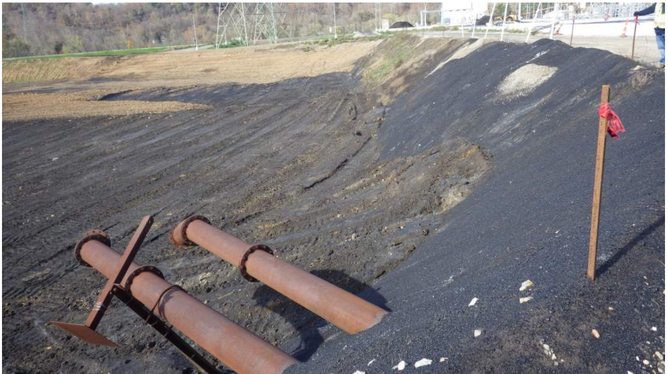
Photograph 18 – Excavation in northeastern corner of boiler slag closure area.
