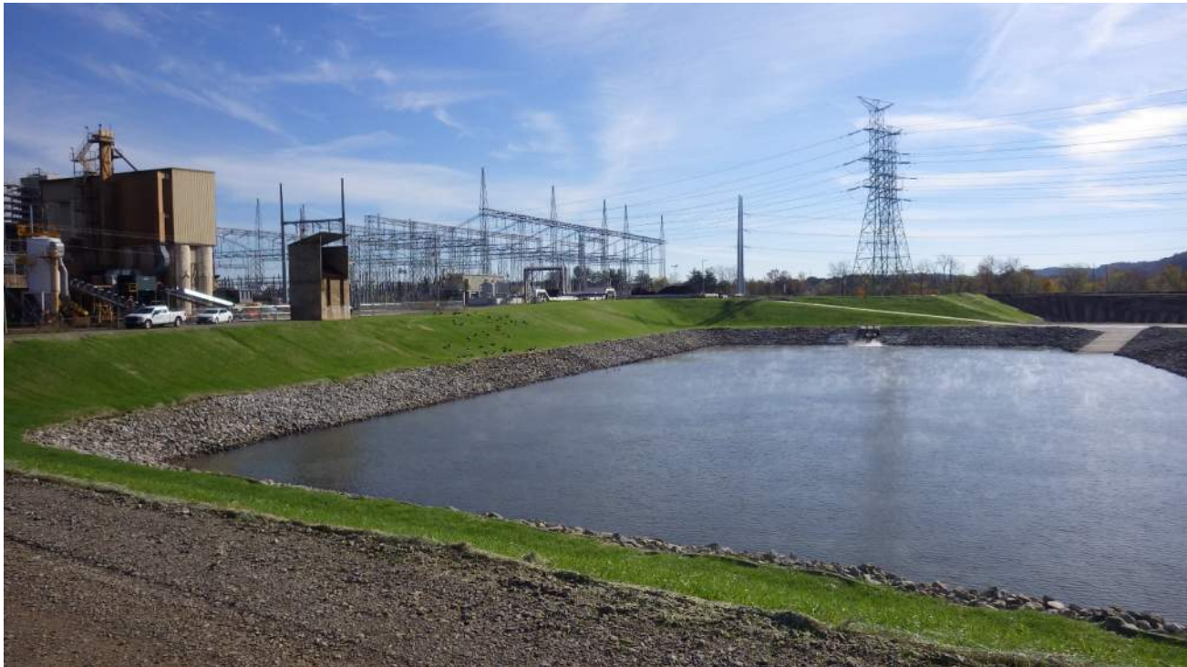
Photograph 3 – New vegetation at northern side of LVWTS, primary basin.
