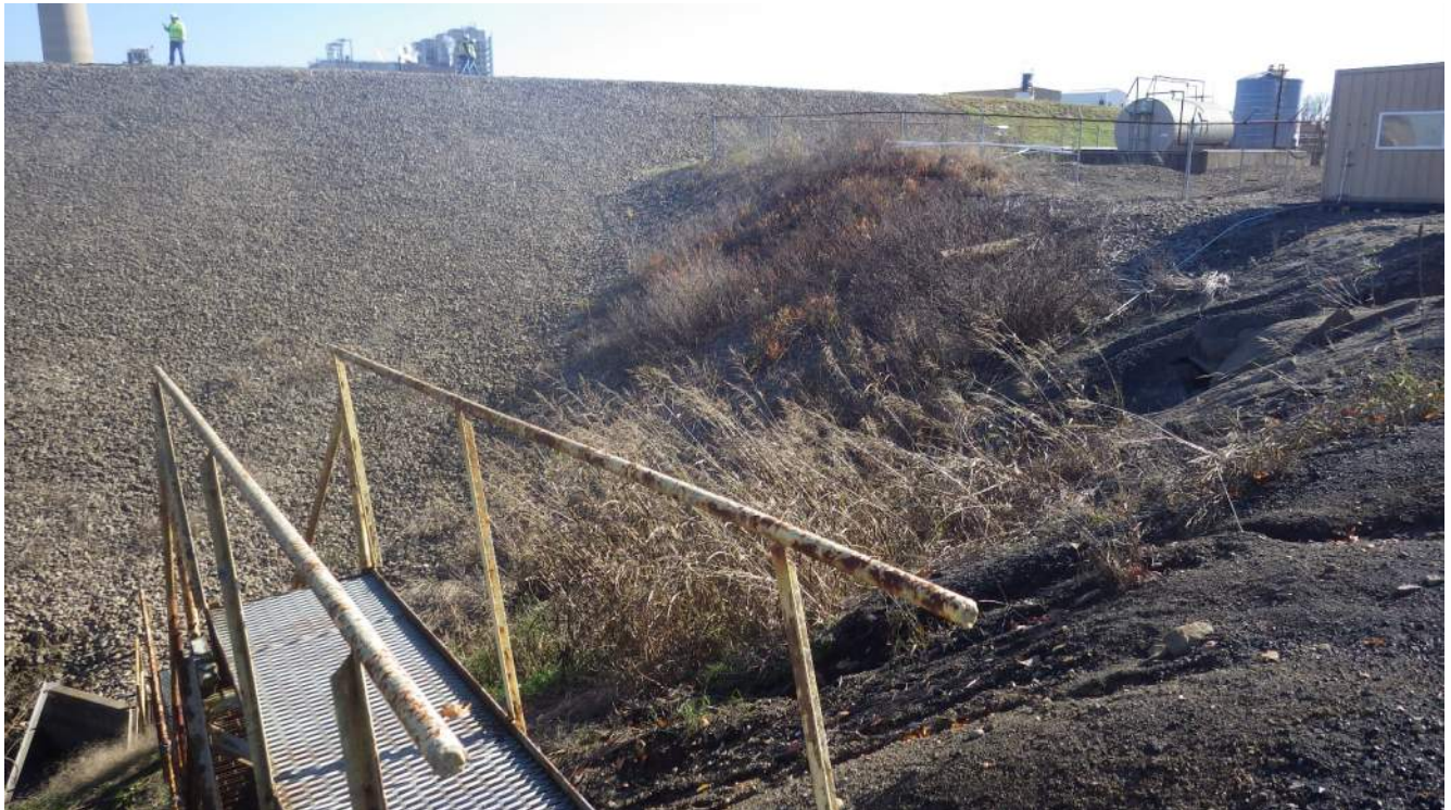
Photograph 14 – Outfall to Kyger Creek west of SFAP.
