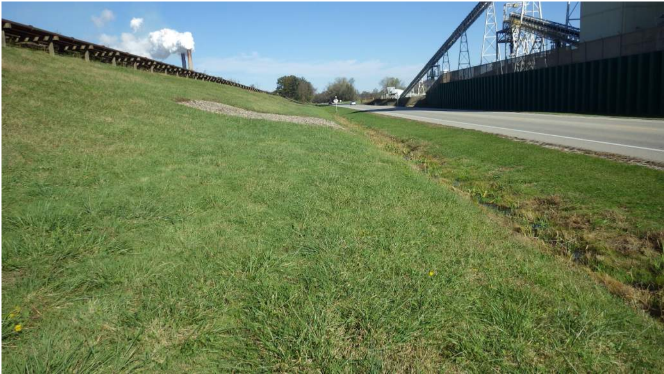
Photograph 6 – Seepage blanket on downstream side of eastern perimeter embankment.
