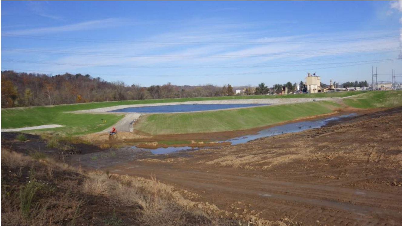
Photograph 10 – BSP water management and pumping adjacent to LVWTS.
